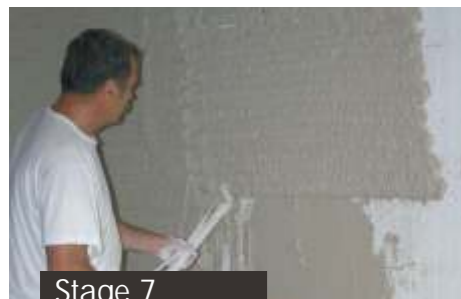
Stage 7 Internal gypsum plaster applied mechanically
