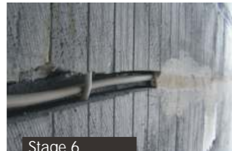
Stage 6 Electrical wiring in grooves
